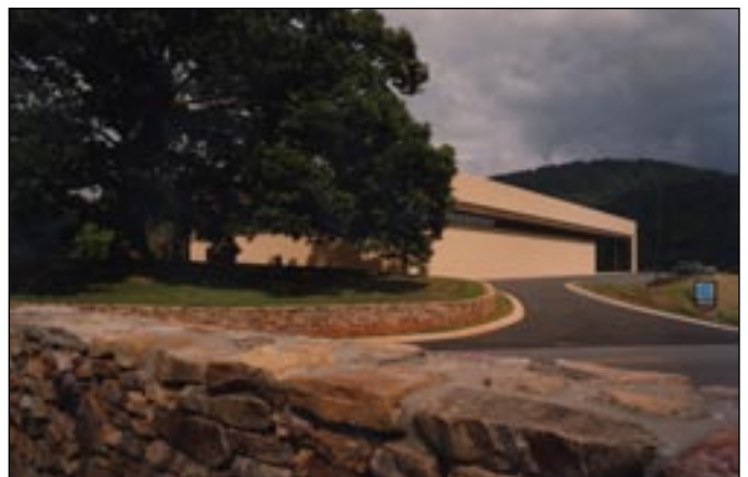
Carolina Conveying Corporate Headquarters located near Beaverdam Industrial Park, Joe Sam Queen, Architect
