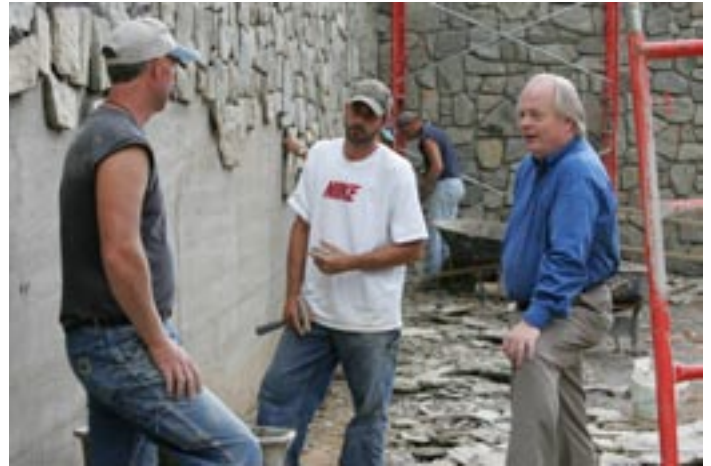
Construction jobs are essential for Western North Carolina.
